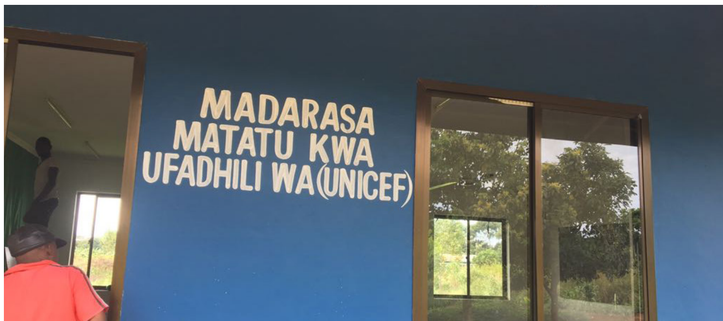
One of the classrooms that UNICEF renovated following the September 2016 Kagera earthquake. Photo| UNICEF Tanzania
