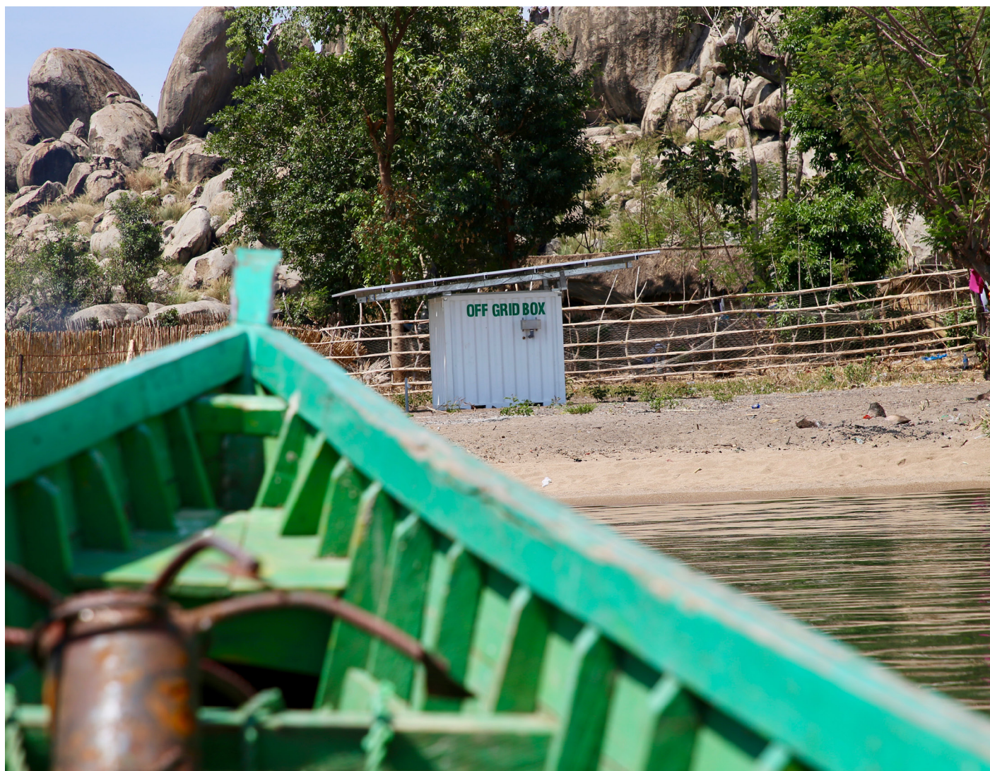
Since Tanzania gained independence, the island of Namuguma in Bunda district, Mara region, has not had access to running tap water. Thanks to the installation of the Off-grid Box, residents are now enjoying access to clean energy and safe water. Photo | UNDP
