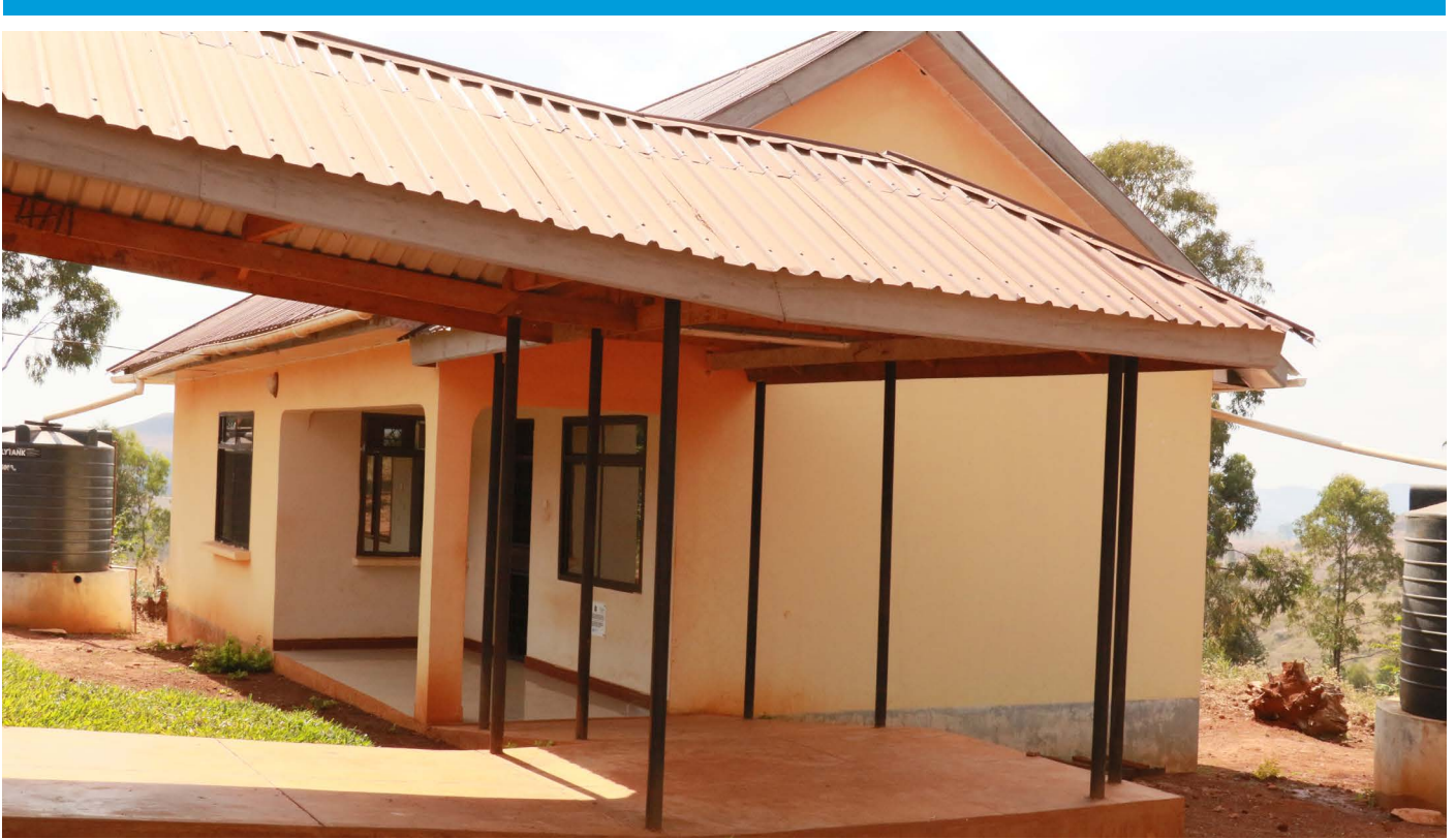
A newly renovated labor ward at the Mwanga dispensary.
