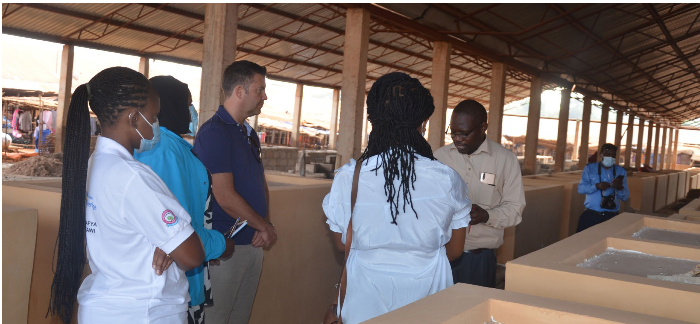
Mr. Adili Mlowe, Planning Officer for Kasulu Town Council, briefing Mr. Matthias Lindström from the Embassy of Sweden on the benefits of the rehabilitation of the Sofya Market. To date, 220 women traders have been provided permanent trading stalls at the market.
