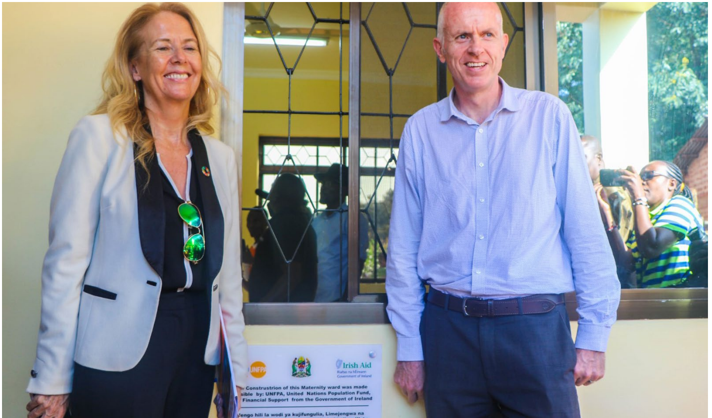
Ms. Jacqueline Mahon (left), UNFPA Country Representative and H.E Paul Sherlock, Irish Ambassador to Tanzania at a newly constructed maternity ward at Muzye village in Kasulu District. The building, which is among 9 wards constructed under the programme will enhance the delivery of quality emergency obstetric and newborn care, both basic and comprehensive in the project districts, including capacity strengthening of healthcare providers.
