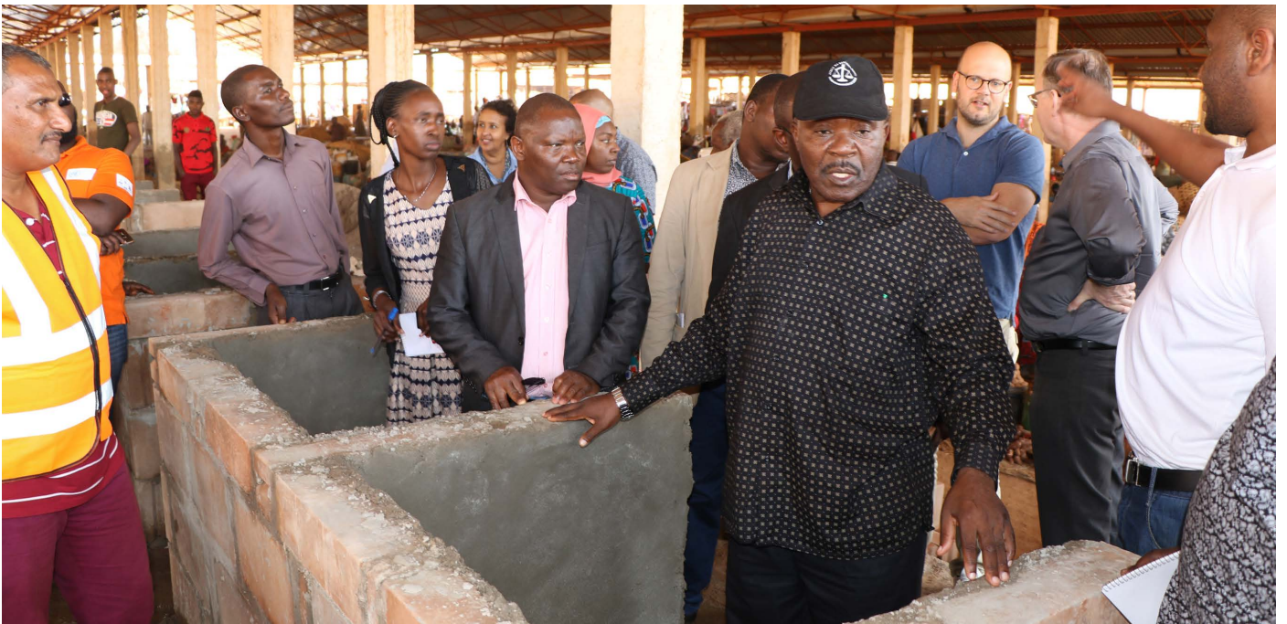
Here the Regional Commissioner is inspecting the new stalls for the traders which are being constructed by the International Trade Centre (ITC). These will be built for the entire indoor section of the market and will feature storage space so that traders have somewhere secure to keep their goods when they close shop for the day.
