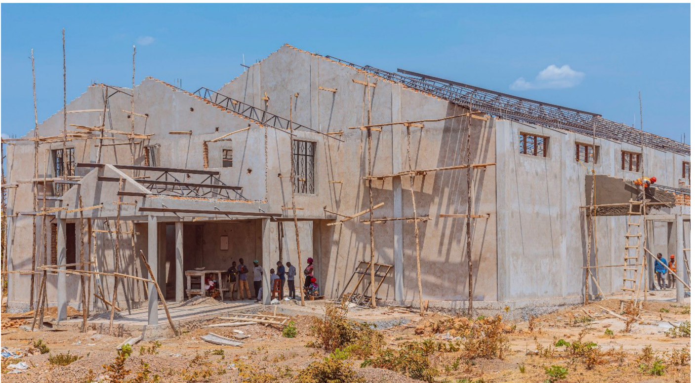
Mvugwe aggregation center under construction. Photo | UNCDF/Mariam Simba
