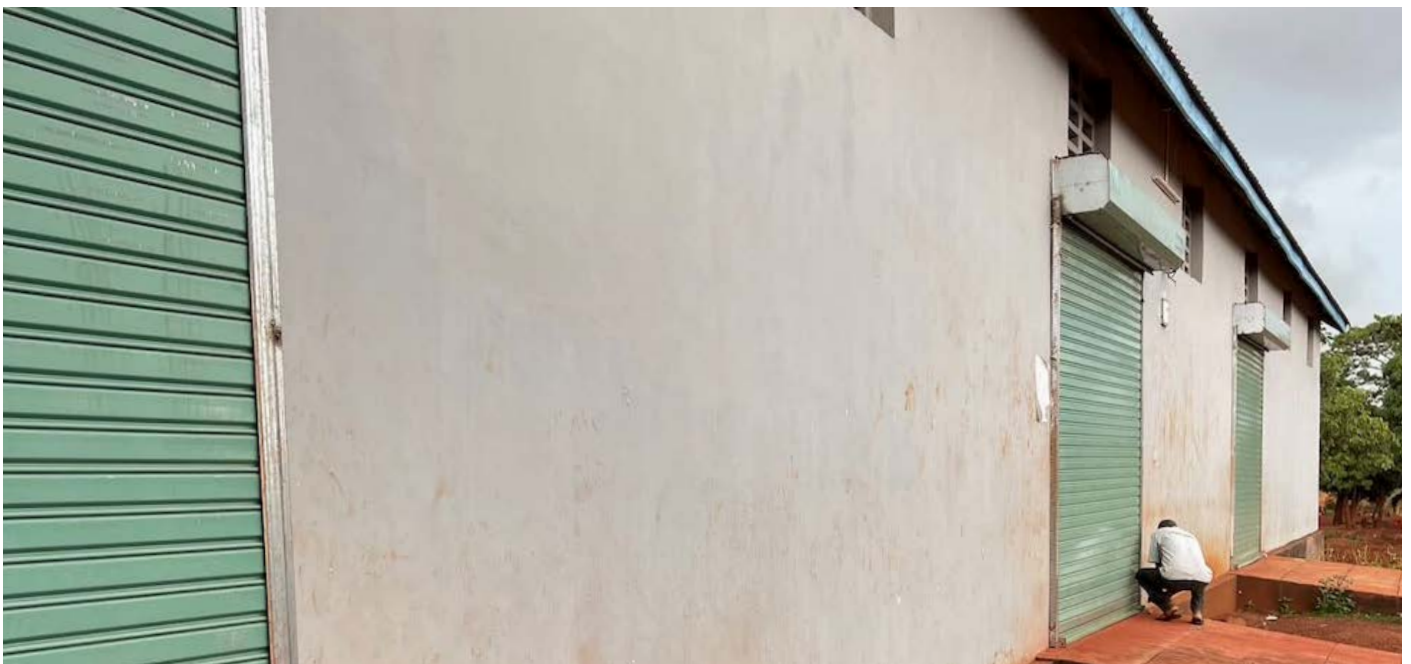
Newly constructed Kabingo storage facility
