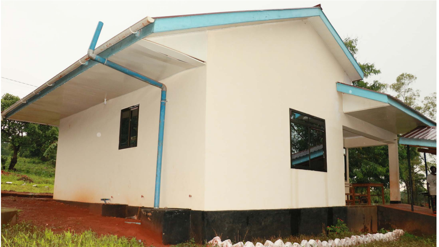
Newly constructed Nyarugusu Maternity ward.
